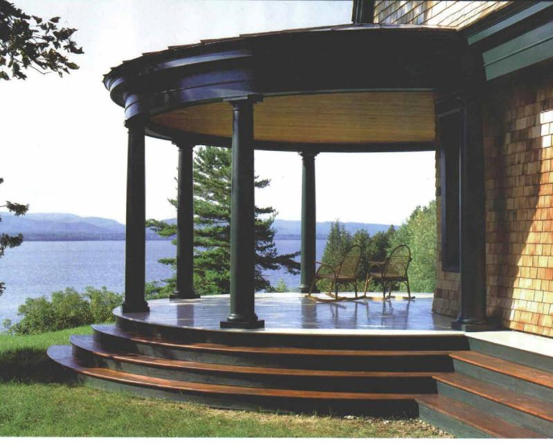
**A few strategically placed columns support the roof.** Because the weight of the roof was evenly distributed on the rigid laminated beam, columns were required only beneath the section joints. The resulting open spans also give room to enjoy the view.
