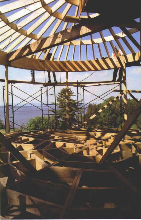
**Building in the round relies on the art of framing.** The floor frame slopes from a central point to shed water and was configured to support a radial pattern of decking. Consistent spans between the rafters above meant plenty of support for the roof sheathing.
