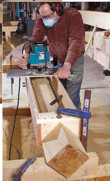
Angled sled turns four sides into eight. A sled similar to the first, except that it's equipped with 45° angle blocks, directs the router to cut the angled sides of the octagon.
