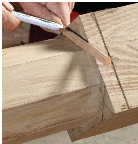
An eight-sided bead as well. A gauge block set at the proper depth marks the angled sides of the bead. The same angled router sled that cut the octagon is repositioned, and the depth of the bit is adjusted to cut the angled bead.
