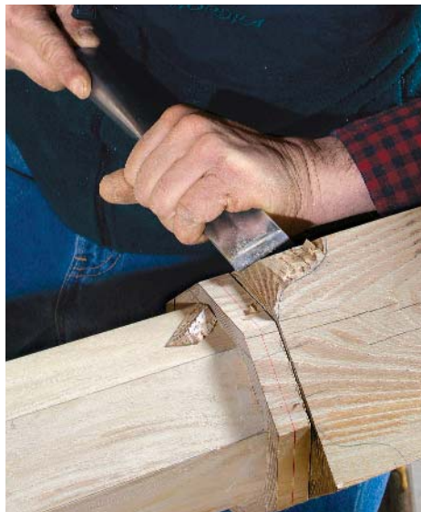
Razor-sharp tools for hand-carved details. To create the carved details at the top and bottom of the octagon, flat chisels pare down the convex surfaces (photo center), and a curve-bladed gouge shapes the concave surfaces (photo right).
